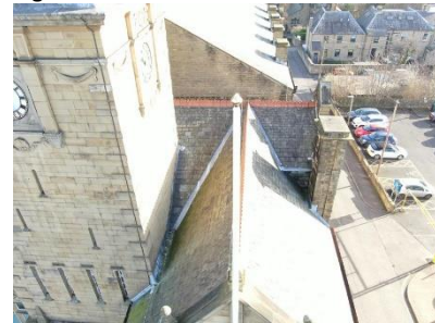
Figure 4 Roof to right side of clock tower
