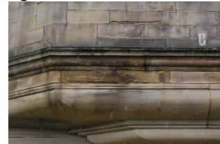
Figure 15 Typical area of repointing and descale
