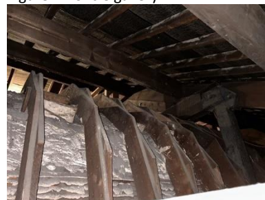
Figure 70 Circle gallery support structure
